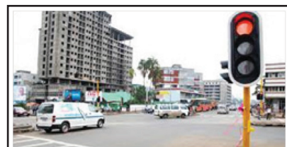
Figure 1.62 - Traffic Lights Control System
